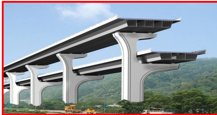
Figure 1 the F-bent double decked bridge column
