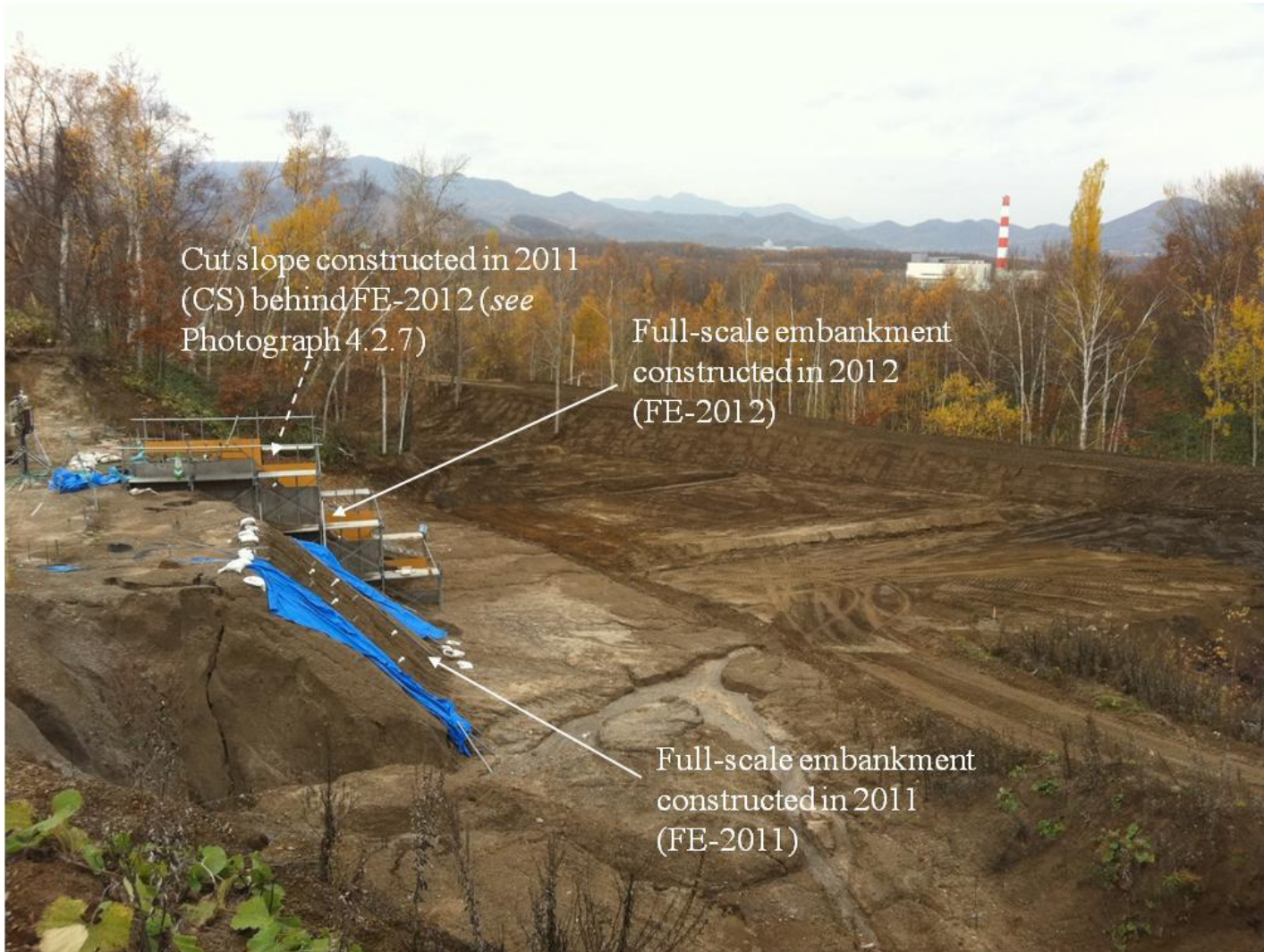
Photograph 4.2.1 Whole view of embankment site
