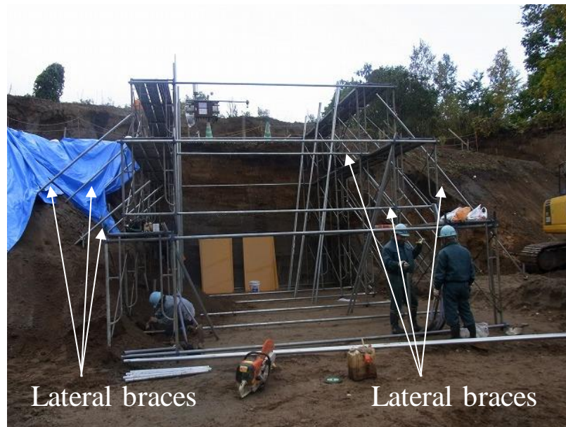
(a) Structuring lateral braces
