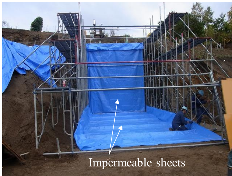
(b) Laying impermeable sheets
