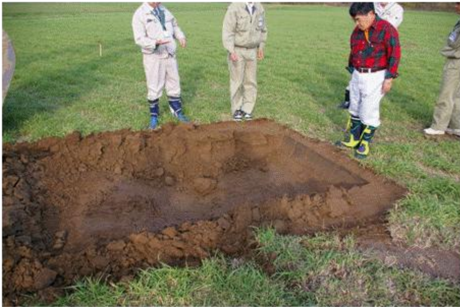
Photograph 3.1.1 Borrow pit for Ikeda sandy silt
