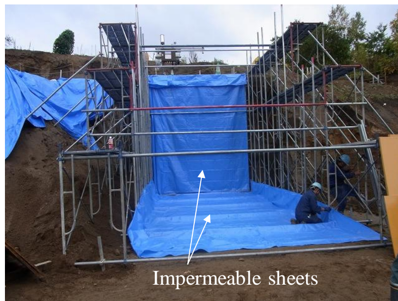
(b) Laying impermeable sheets
