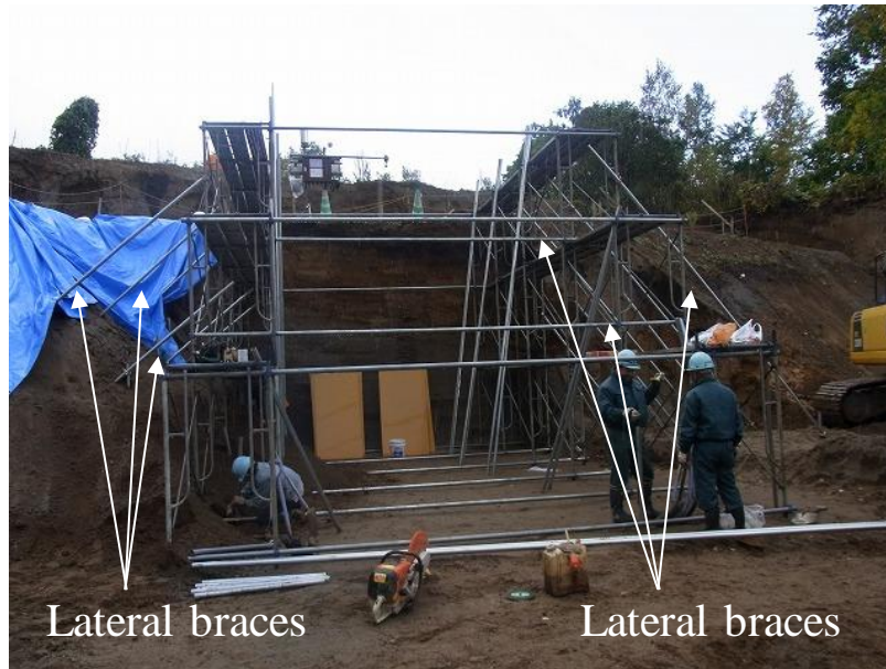
(a) Structuring lateral braces
