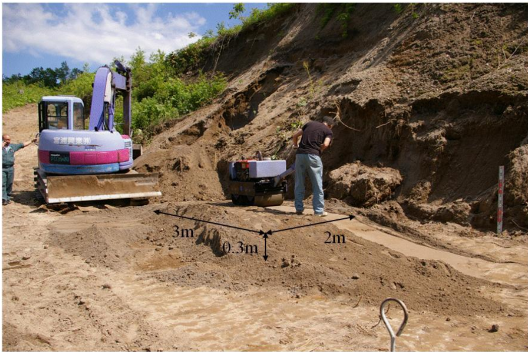
Photograph 4.2.3 Trial construction on 2011.06
