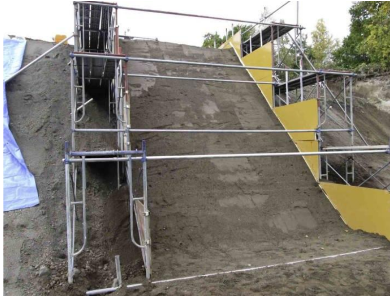
(g) FE-2012 completely constructed
