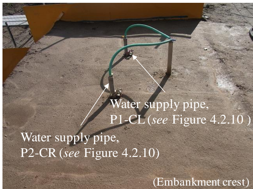
(h) Water supply pipes
