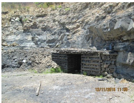
Figure 2: Mine adit with well constructed canopy at Mean- Jalawe Coal Mine
