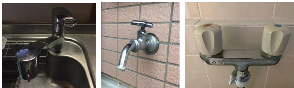
Fig. S1 Examples of taps (left: single-lever mixer tap; middle: standard tap; right: double-handle mixer tap)
