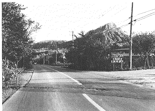
Photo. 1. Dislocation of the road at Point A in Fig. 4 (a). (photo. Sept. 1978)
