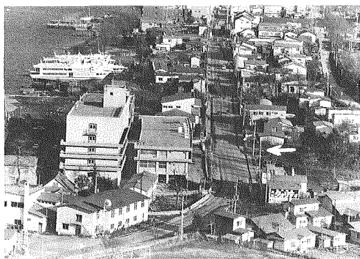
Photo. 3. Dislocations of the road and a building at Point C in Fig. 4 (b). A white arrow indicates a fissure line. (photo. Nov. 1978)
