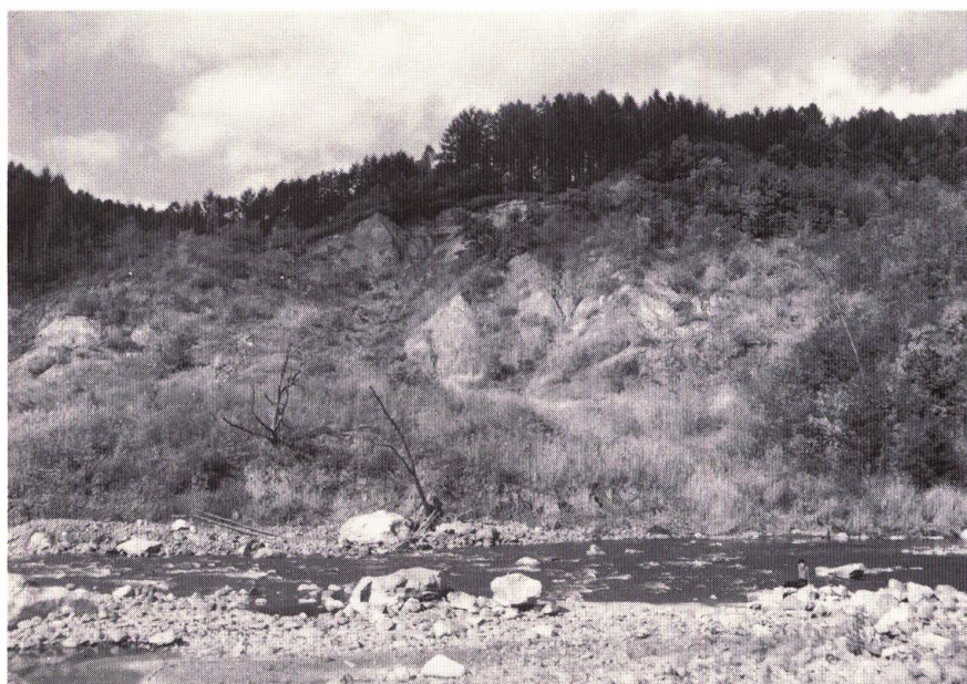
Photo 2. Large accumulation of landslide debris in the foot slope (Saru River).
