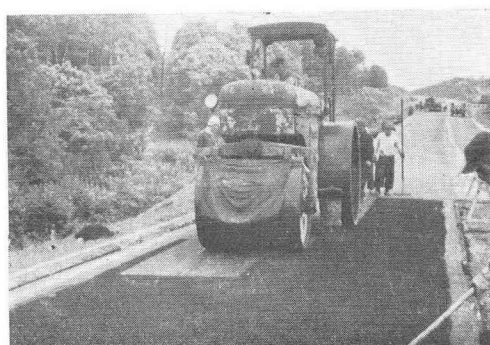
Photo 2. Placing and rolling of rubber blended asphalt mortar in the test road section.
