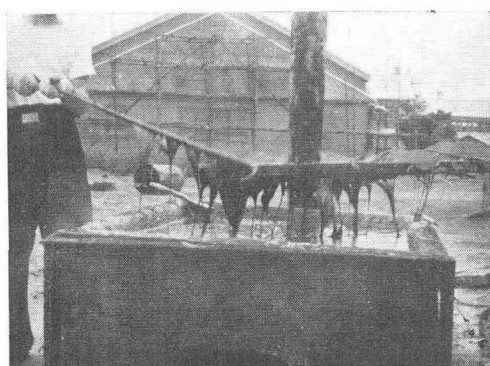
Photo 1. Rubber blended asphalt cement in a kettle.
