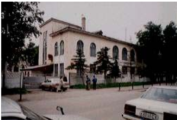
Fig. 15. The Karafuto-Cho Annex Building (1934)
