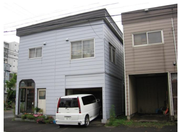
Fig.5. The very narrow open spaces between the houses would still provide daylight and access to some services.
