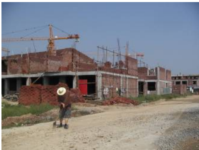
Figure 2.1 Construction site of S village
