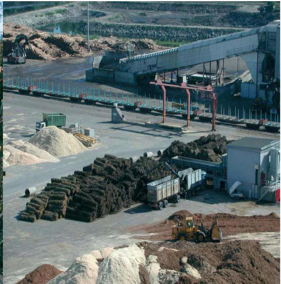
At the power plant
