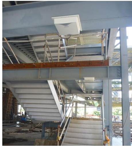
Figure 2: Installed RFID devices in the construction site.
