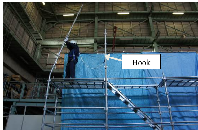
Figure 10: The worker who tried setting other supports.
