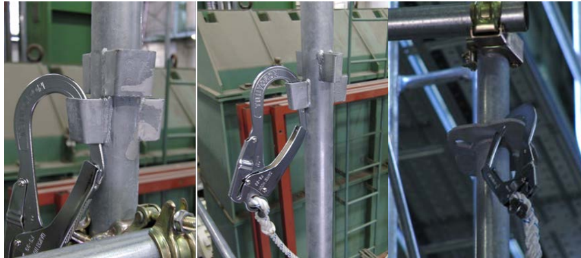
Figure 3: Typical wedge pockets and the hook of the safety harness (Left: Type A, Center: Type B , Right: Type C).
