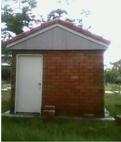
(a) the interlocking block room
