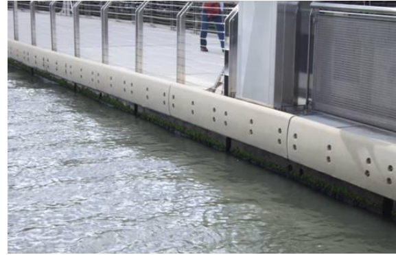
Figure 5: Fibre composite reinforced waler
