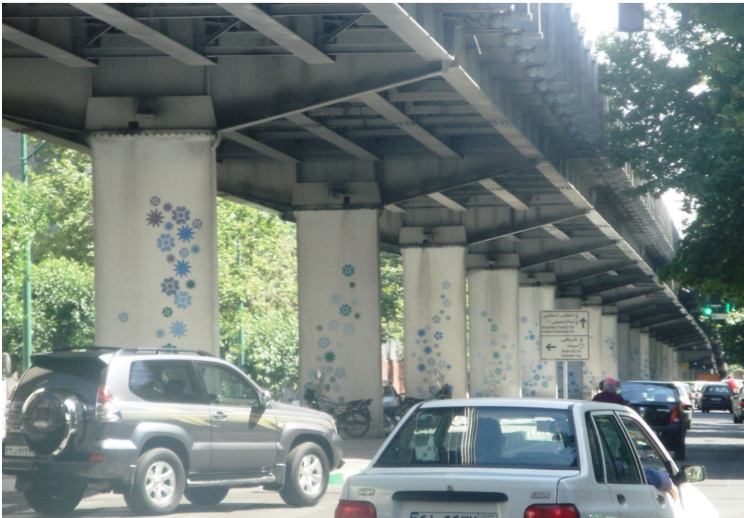
Figure 1: A general view of the considered cantilever pier type overpass bridge
