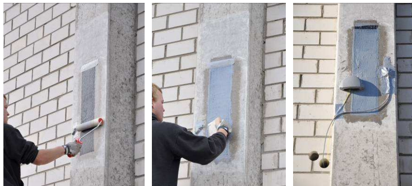
Figure 5: Handling at building site.
