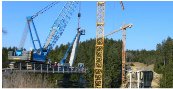
Figure 5: Vertical assembling of the arch
