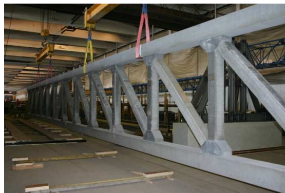
Figure 7: Truss construction for the full scale test
