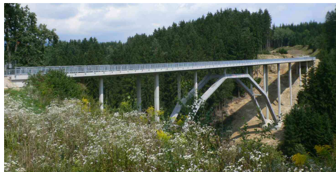
Figure 1: The road bridge Wild
