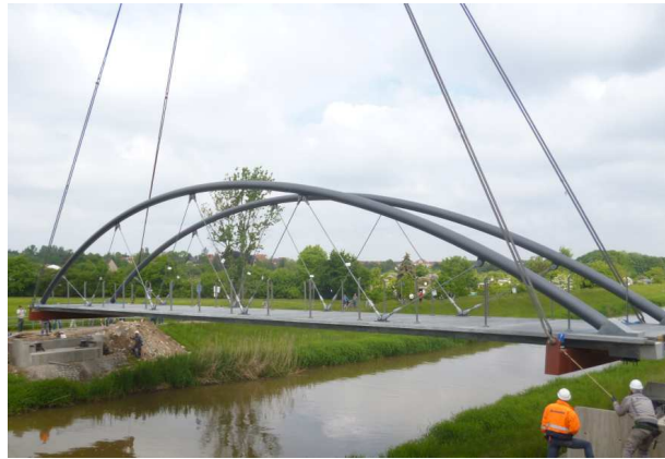
Figure 11: Assembly of the bridge with mobile crane
