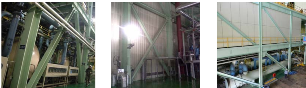
(a) Inverted V-Brace
