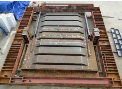
Figure 5: Assembling of prestressing table and deck form.
