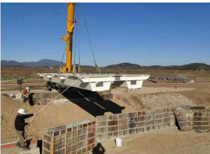
Figure 8: Erection of U-girder.
