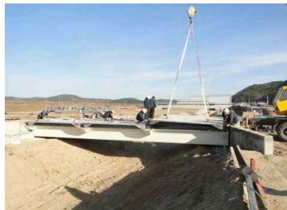
Figure 9: Erection of deck panels.
