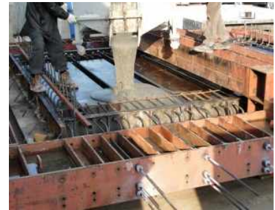
Figure 7: Placing of UHPC.
