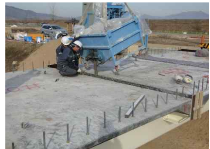
Figure 10: Placing of UHPC joints.
