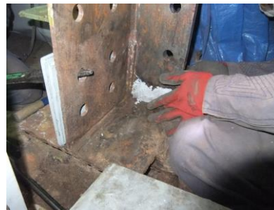
(a)Gluing epoxy resin
