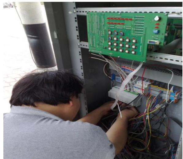
Picture 5.2 the Installed Traffic Controllers at the Intersections
