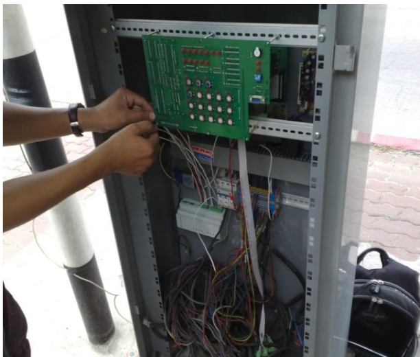
Picture 5.2 the Installed Traffic Controllers at the Intersections
