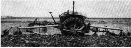
Fig. 1.2 “Agri-Robot”, unmanned plowing robot
