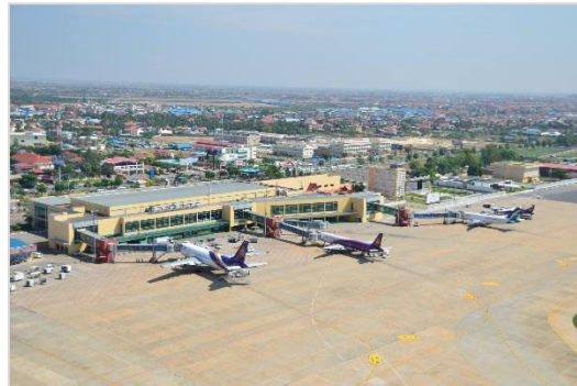
Figure 2-12: Phnom Penh international airport
