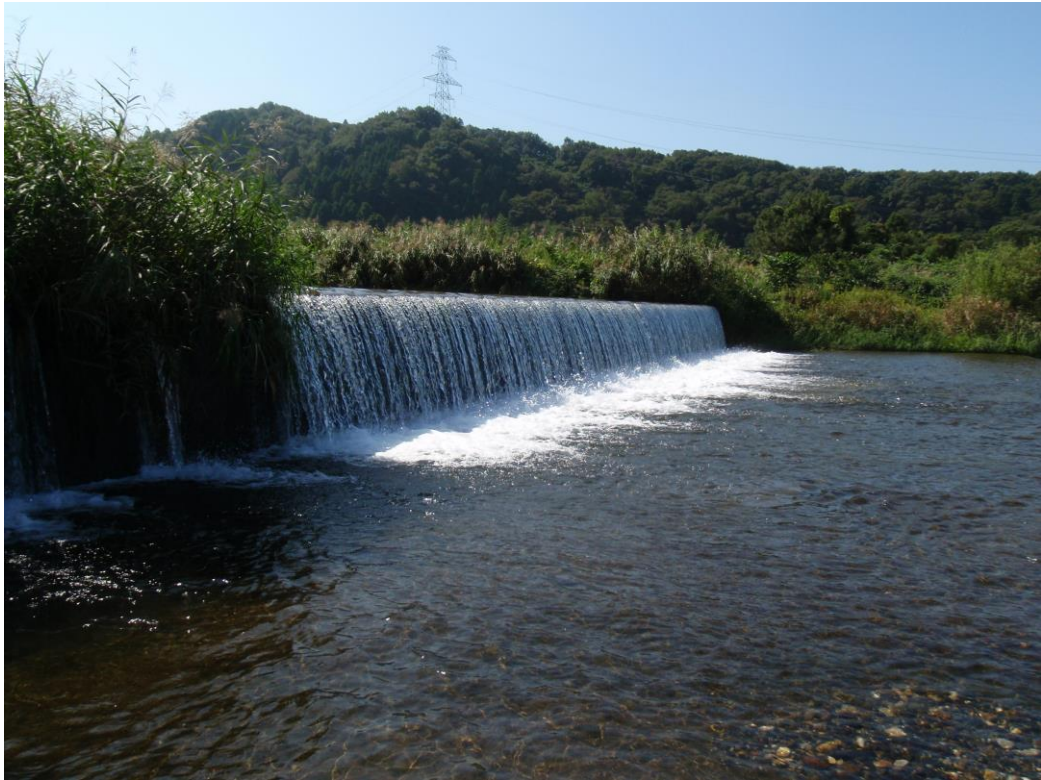
Fig.6-1. Low dam: prevent upstream migration of Biwa salmon in the Ane River.
