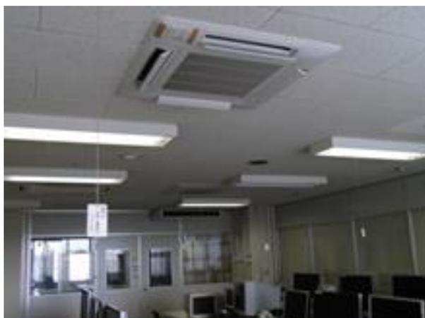
Fig. 6.11 Indoor units of conventional system (back) and developed system (front) at Shizuoka (Hitachi-Johnson Controls Air Conditioning, Inc.)
