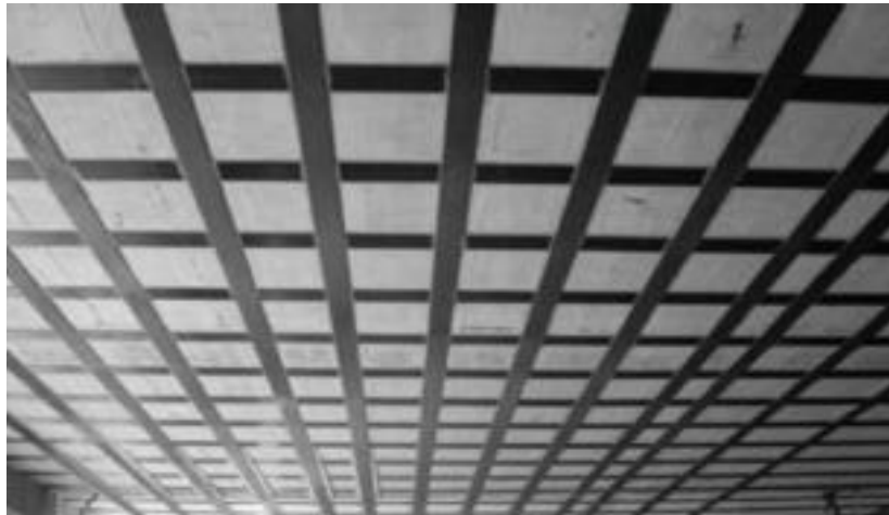
Fig. 1.3 CFRP strengthening
