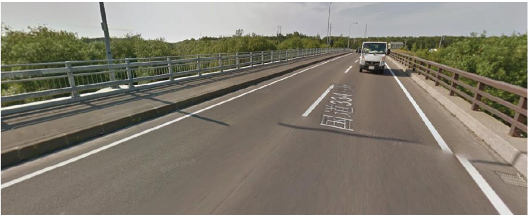
Fig. 1.2 Shuen-Bridge (National Highway Route 334, Shari, Hokkaido, Japan)
