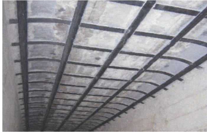
Fig. 2.15 Strengthened RC slab
