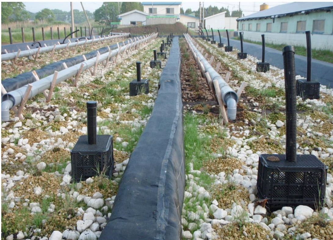
Fig. 2-3 Surface partition and reinforced safety bypass.
