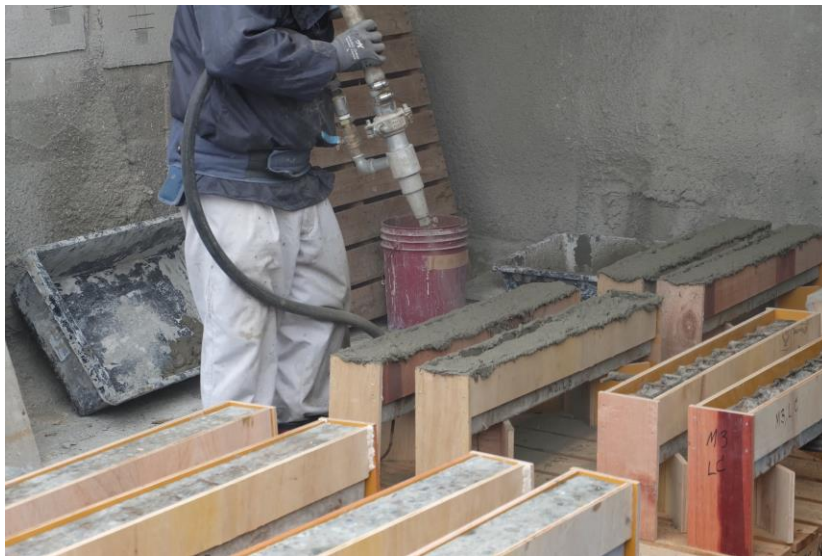
Figure 3.5: Spraying polymer cement mortar
