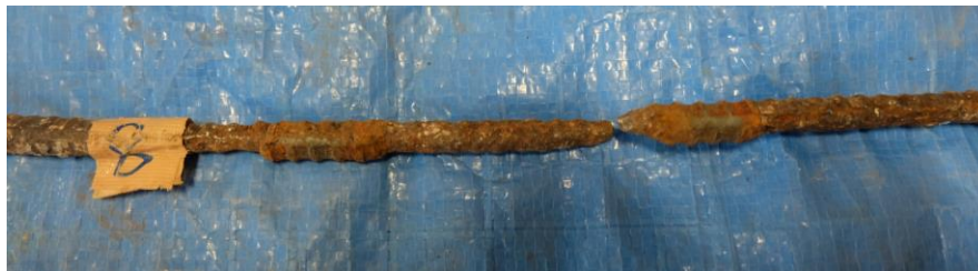
(b) Steel bar corrosion for the beams in group 2
