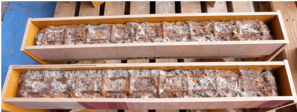
(b) Repair method 2
