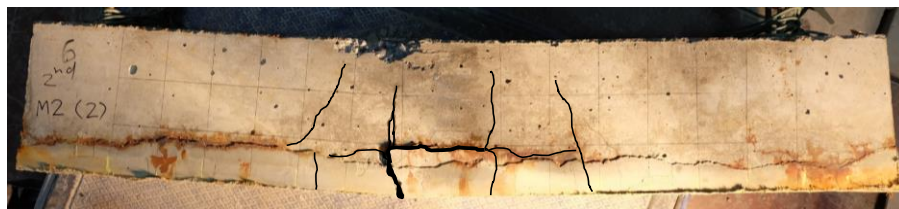
(a) The beam repaired with method 2
