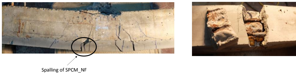
Figure 3.17. Spalling of non-fiber containing SPCM
