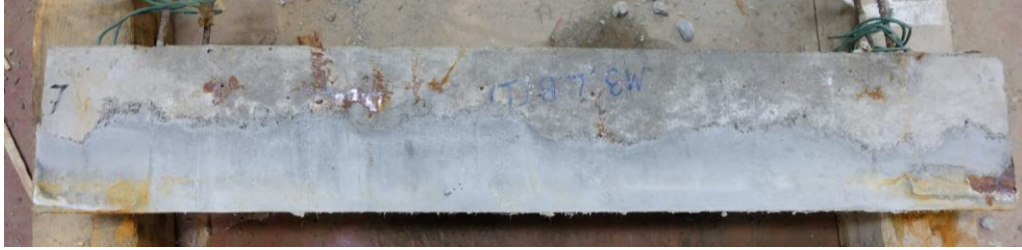
(b) After finish corrosion for the second time
