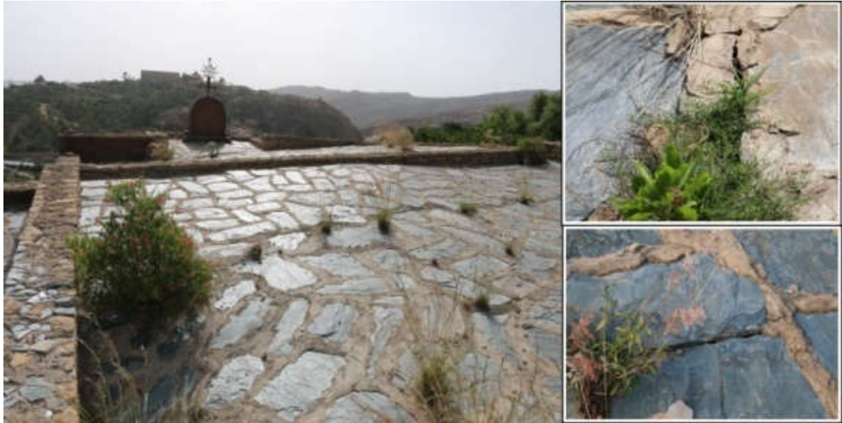
Fig 4.23. Flagstone roofing, Wukro Cherkos, 2016
