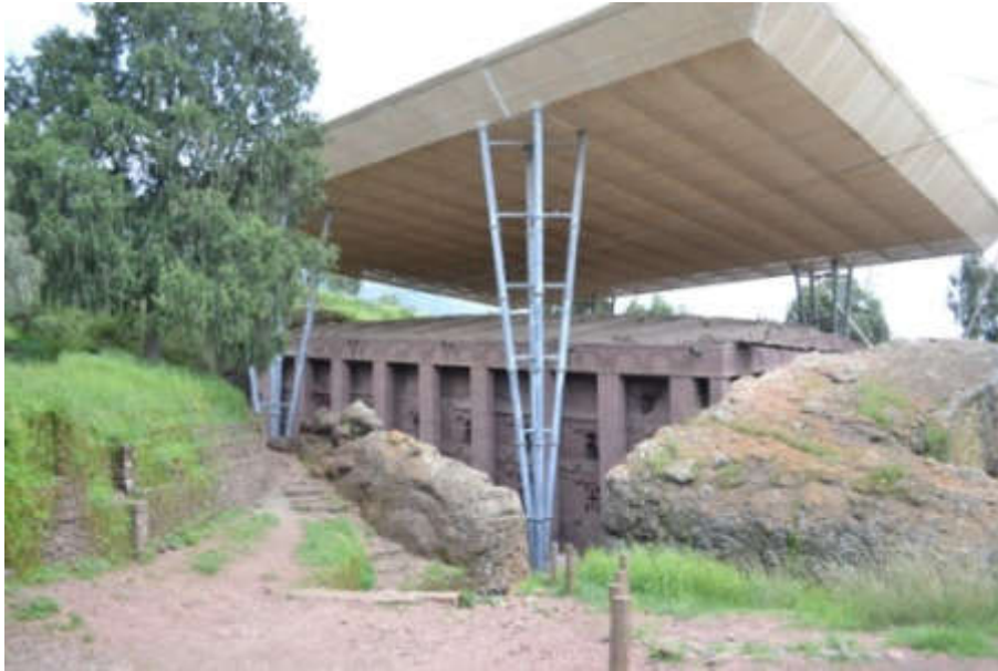
Fig. 4.34 The realized shelter
