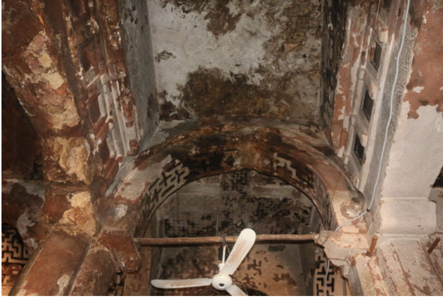
4.3 Ceiling of Abreha we Atsibeha Church
