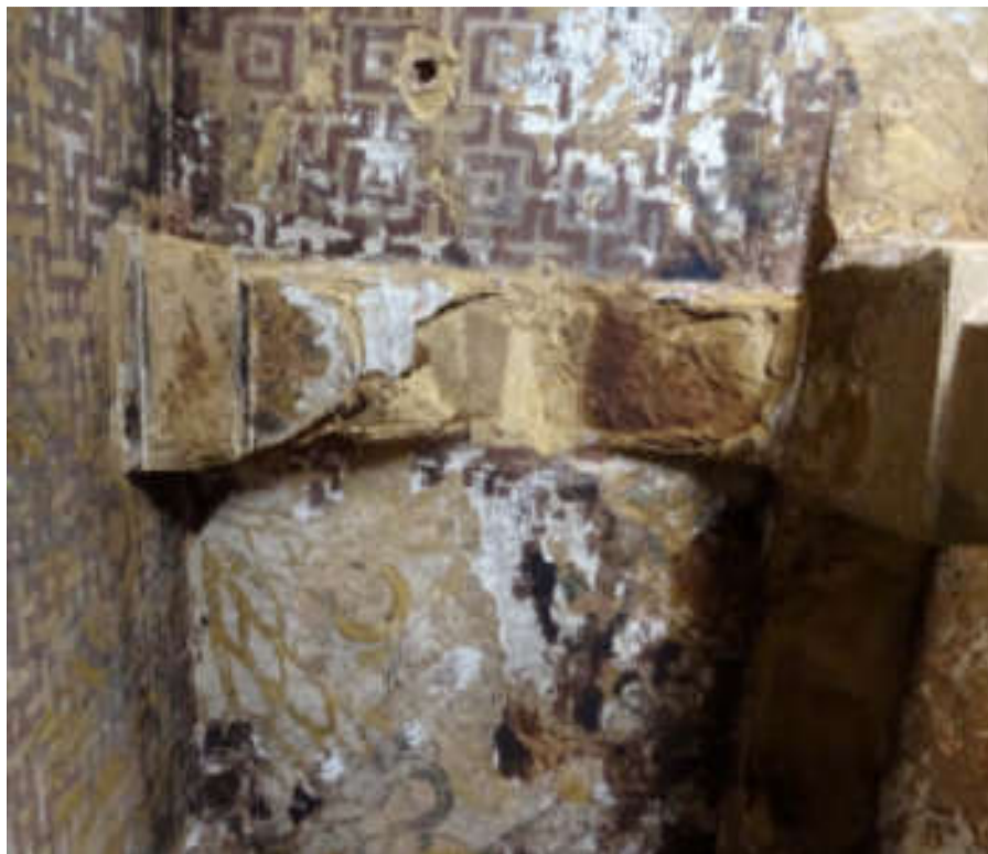
Fig 4. 25. Mould growing in the ceiling and a n arch falling apart
