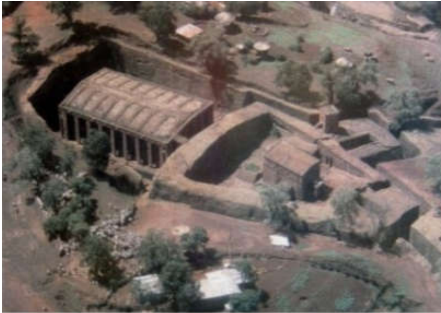
Fig. 4.30 Bete Medhane Alem after the restoration of 1967
