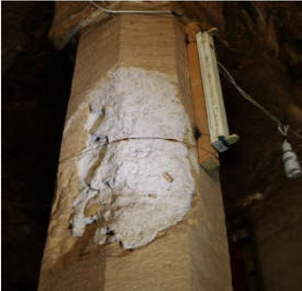
Fig 4.22. A column with Gypsum maintenance
