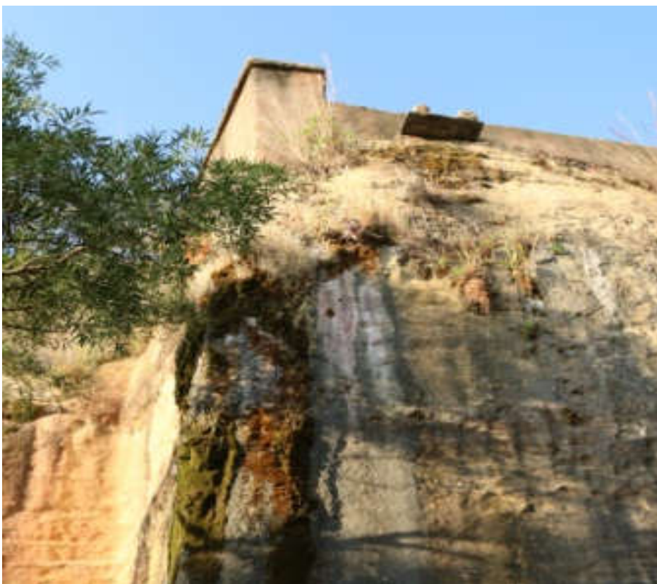
Fig 4. 27. Algae blooming, grass growing and mould in on the exterior wall
