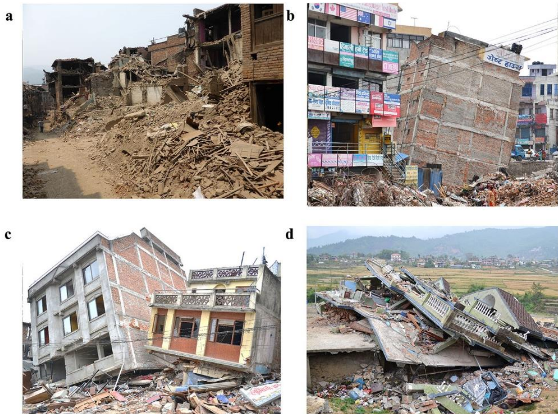
Figure 3. 21 Damage to buildings in a) Bhaktapur, b) Gongabu, c) Sitapaila, and d) Ramkot.
