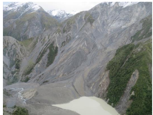
Fig. 1 Landslide dam on the Hapuku River
