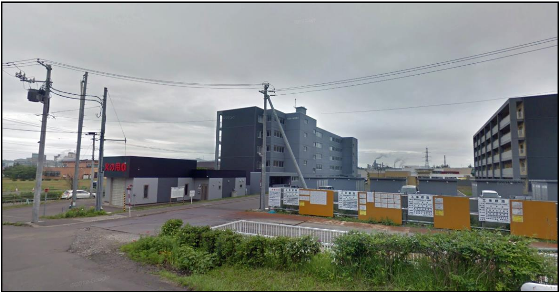
Photo 4-5 Exterior photograph of Nakajima estate
