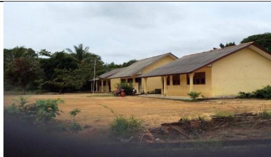
The only elementary school available in Selindung. Its renovation was supported by Suction dredging company (Field Research, Selindung, 2015)
