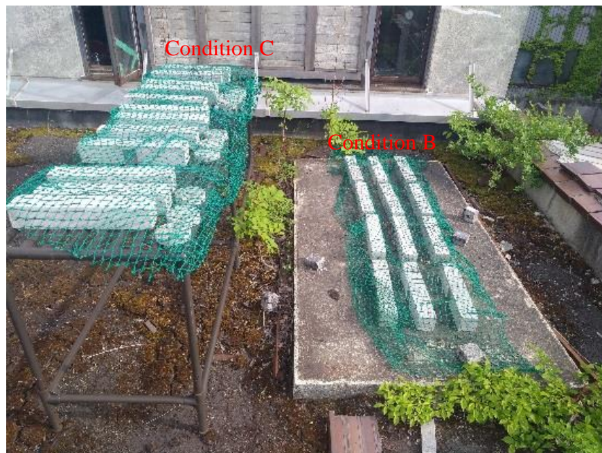
Fig.4.1 The curing condition B and C
