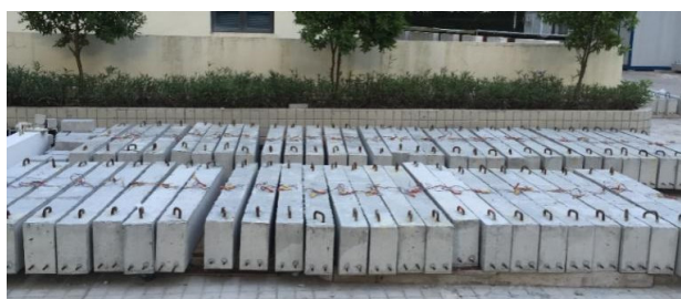
Fig. 2.14 RC beams curing outside atmospherically.
