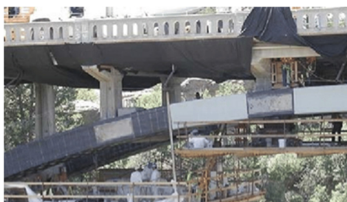
Fig. 1.2 Strengthening of a concrete bridge with CFRP sheet (Sonnenschein et al., 2016).
