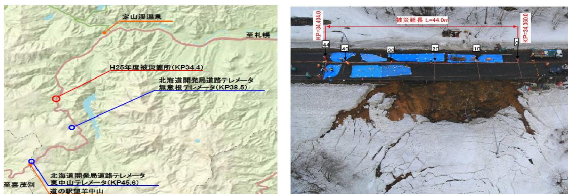
Figure 2.6 (a) Location of slope failure (b) slope failure covered with snow.
