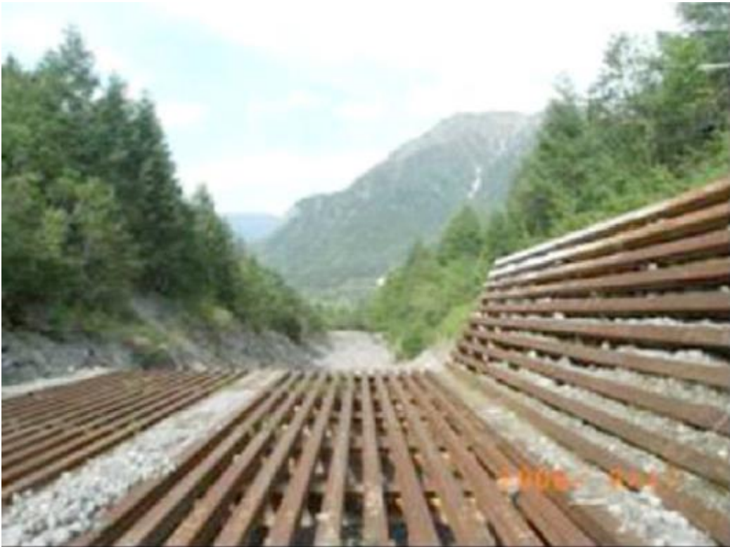
Fig. 6-1. Debris breaker with side breaker ( Brunkal and Santi, 2016 )
