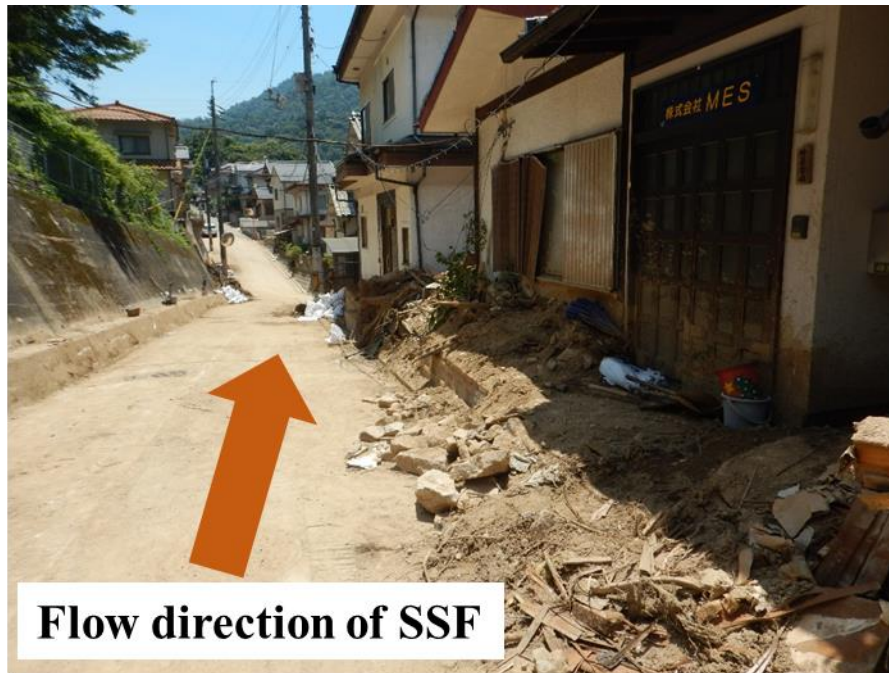
Fig. 1-4. Trace of damage from SSF
