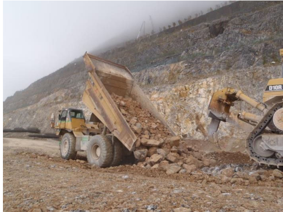
(b) Haulage of limestone from mining area for construction work.
