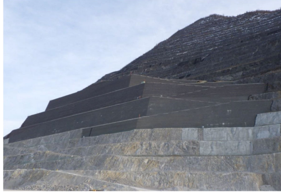
(a) Overall view of retaining rock piling (height of 920 to 990 mL).
