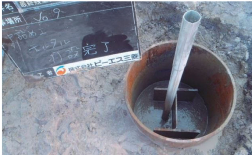
図 4 - 7 Picture of a deep steel piling after completion of cementing.
