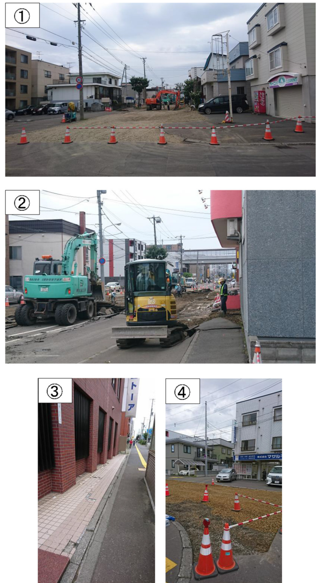
Fig. 15. Damage situation near Kita 34 Station two days after the earthquake (photo locations referred to Fig. 14).
