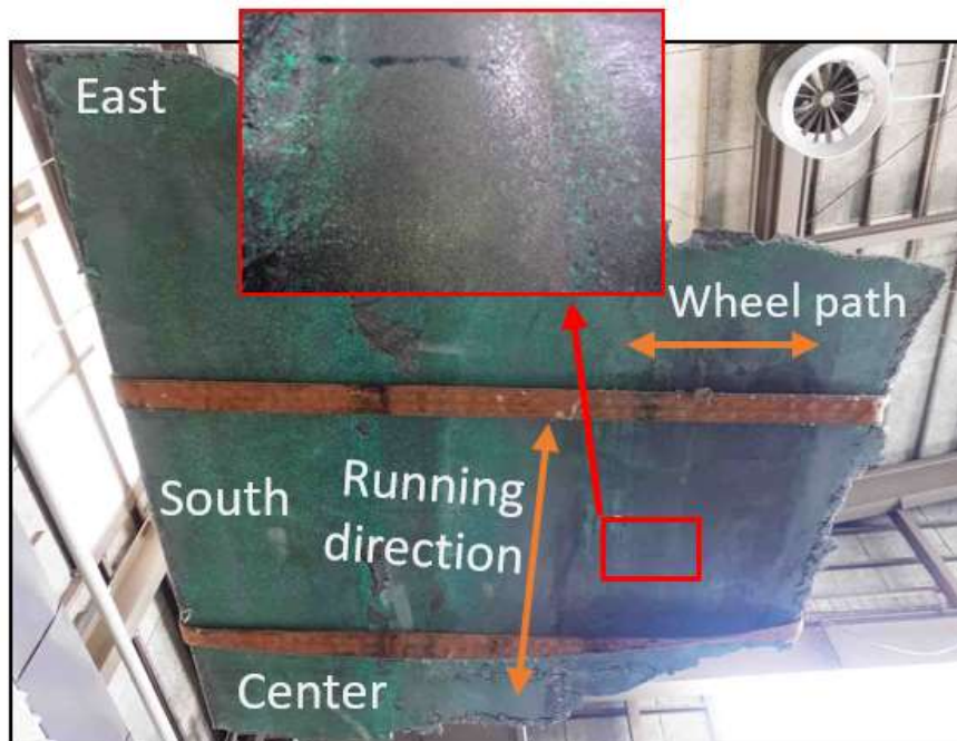
Figure 4.6 Interfacial bond layer under bottom surface of removed UHPFRC overlay at the end of stage 3 from fatigue test.
