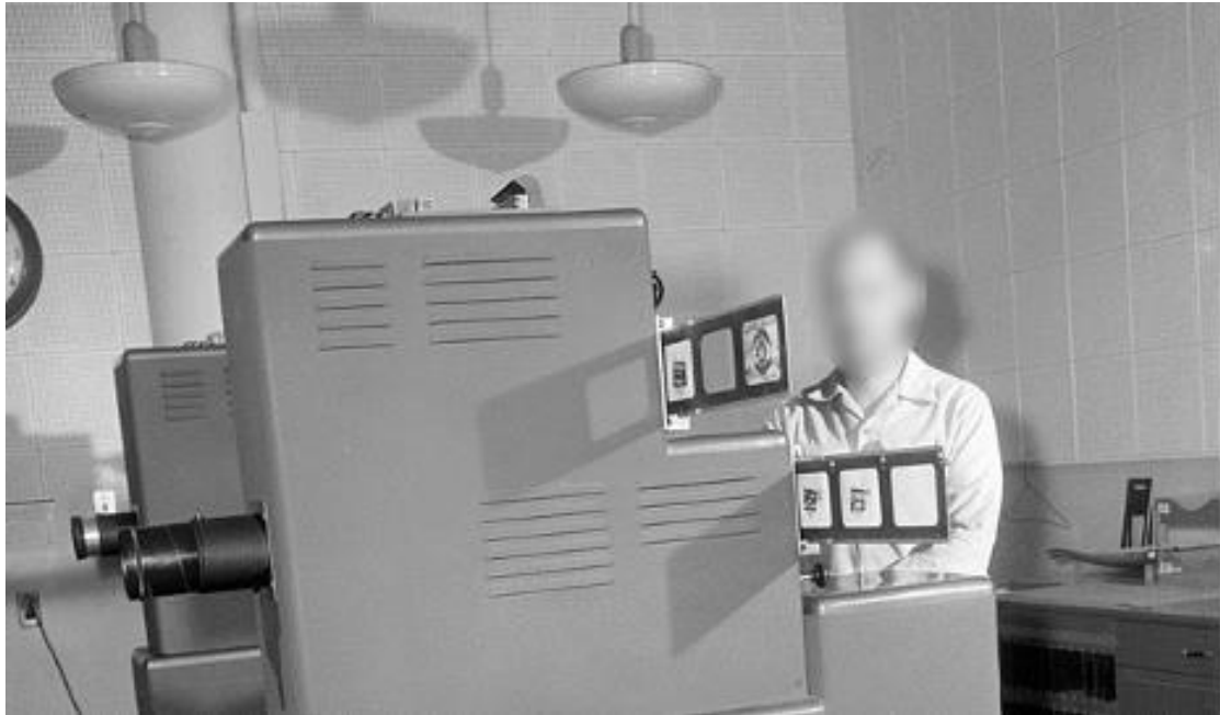
Fig. 2 | Gray Research Telop Machine, Television's First Optical Projection System. This machine was able to televise opaque cards, which was the forerunner of transparent slides. It also had added on features that would allow a news type horizontal ticker scroll across the bottom of the screen (on real ticker tape) and a vertical scroll for credits. The copyright of this image and its descriptions belongs to the person or group with rights.
