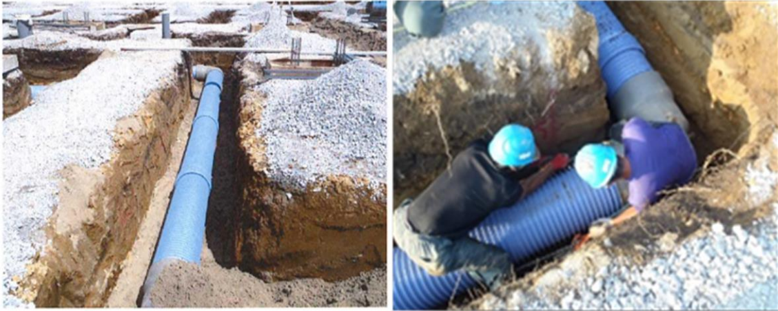
Fig. 6. 21 Figures of earth tube system on construction site
