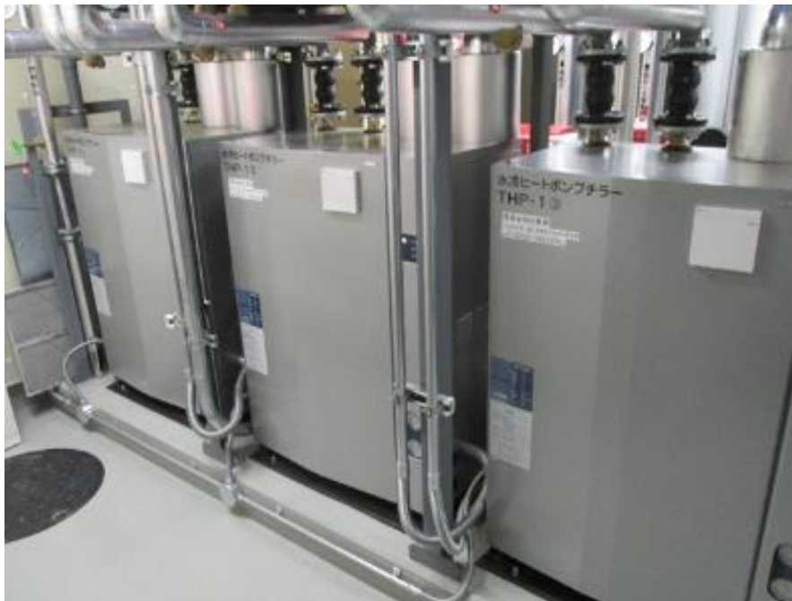
Fig. 6. 20 Figure of the ground source heat pump
