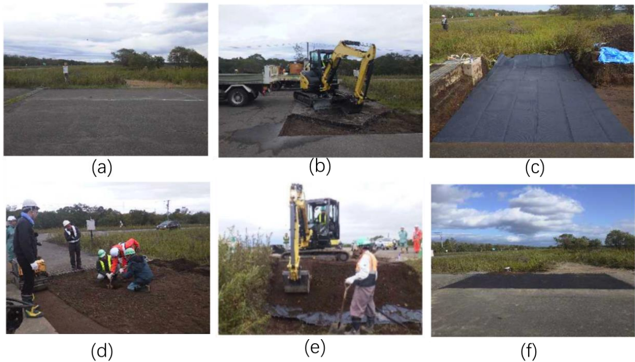
Figure 6.3 The construction process of installing WF.
