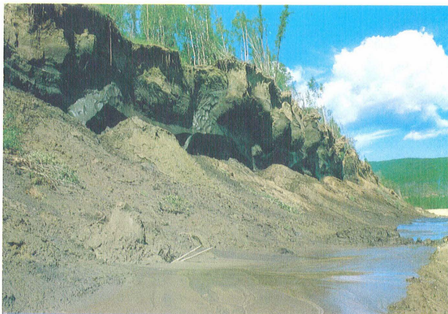
Photo. 1 Underground ice exposed by cutting a road near Fairbanks.
