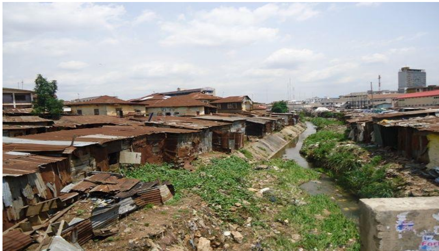
Figure 1.7 Slums in the commune of Kaloum
