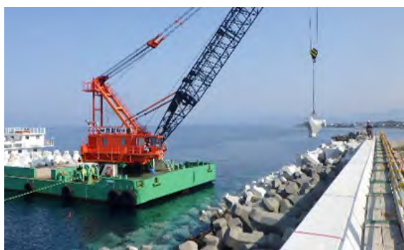
Figure 1.4: Regular supplementary works are required to maintain the height of the stack of blocks.
