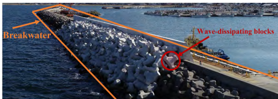
Figure 1.2: Breakwater with its units—wave-dissipating blocks.
