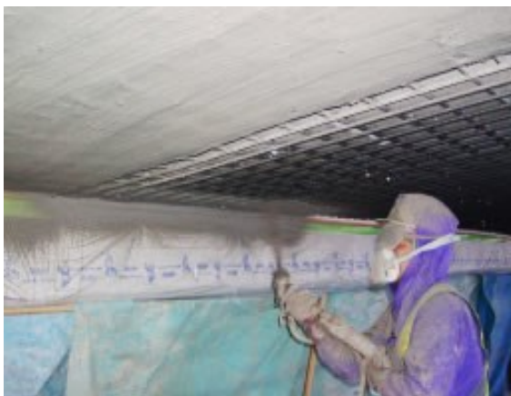
(a) Spraying [Nara Construction Co., Ltd.]
