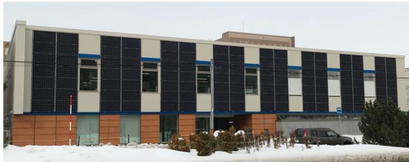
Fig.3-13 South view of the office building
