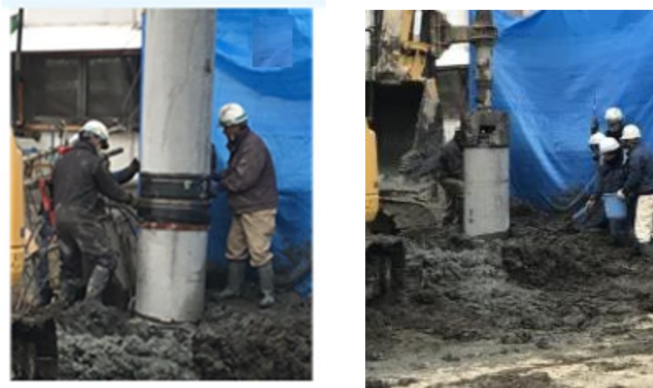
Fig.1.19 Installation process from the construction site.
